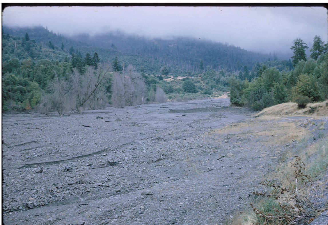
View up Cuneo Cr. from its junction with Bull Cr. Slide taken from the road at N end of the bridge. August 1968
